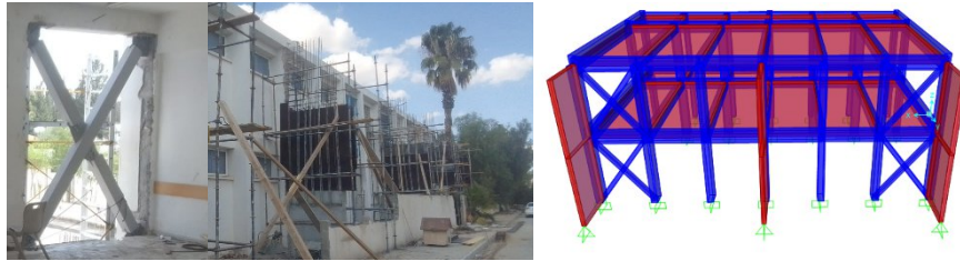
Figure 3. a) Tube 200x200x12.5 X-braced frames, b) 25 cm shear wall, c) Rehabilitated building (Block A)
