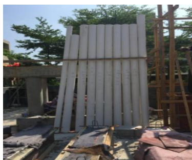
(a) Pipe formwork
