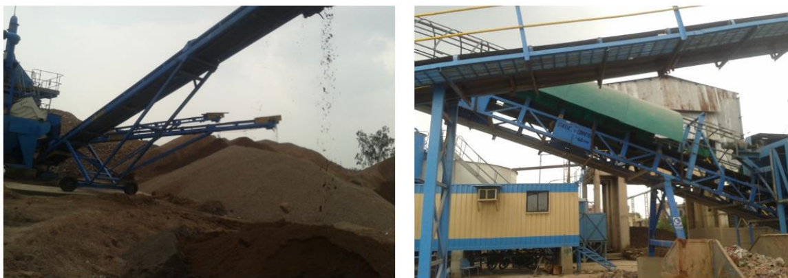
Fig -1: C&D Waste Plant at Delhi, India
