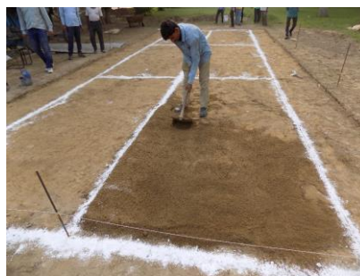
Figure 3: Sub-base layer
