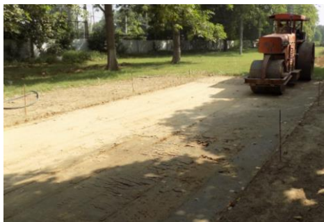
Figure 2: Compacted natural soil used as subgrade
