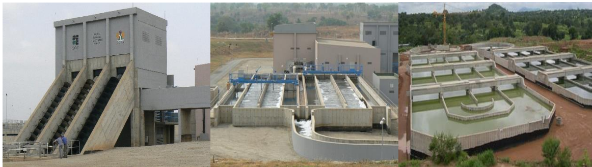
Fig -1: Wupa Wastewater Treatment Plant
