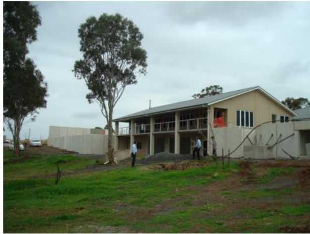
Fig - 13: Precast geopolymer retaining walls for a private residence [43].
