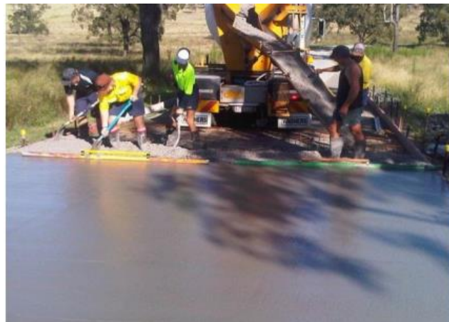
Fig - 12: “Placing of pavement using geopolymer concrete” [43].
