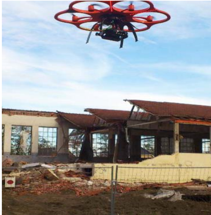
Fig. 3: UAV-based Camera for Structural Damage Assessment [19].
