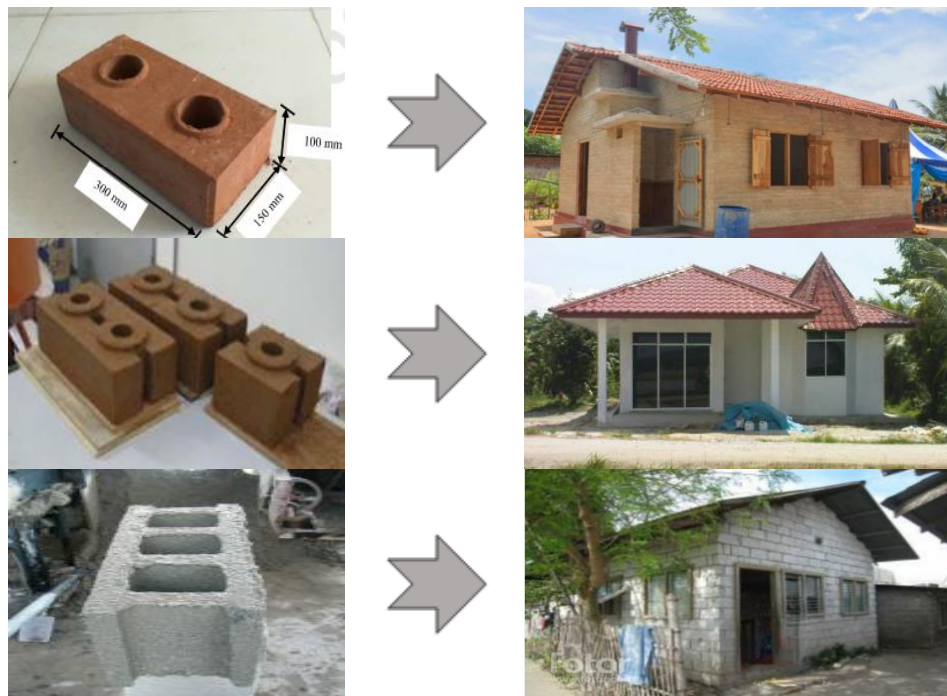
Fig -1: Full-scale houses constructed using hollow blocks; (a) Thamboo et al., (18), (b) Nasly and Yassin (19), (c) Imai et al., (20)
